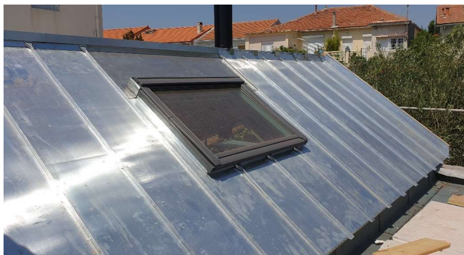
Couverture Joint debout ZINC
